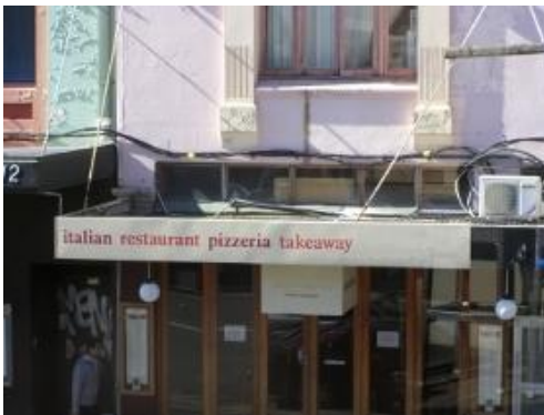
ABC attached above awning on shop front in inner Sydney
