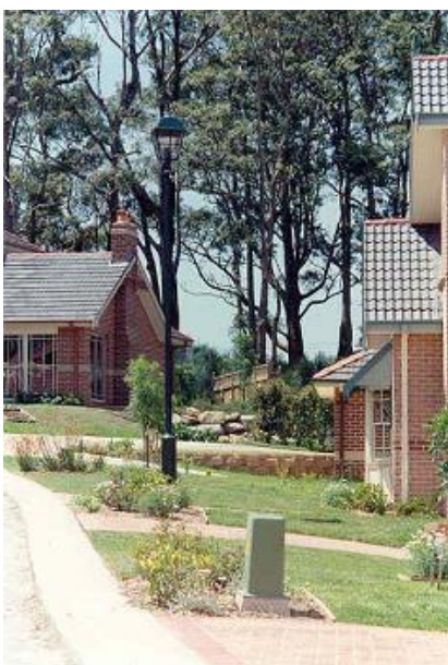
Photo courtesy of Ausgrid
