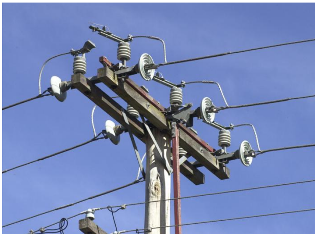
33 kV polymeric post insulator
