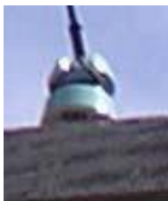
Low voltage insulator
