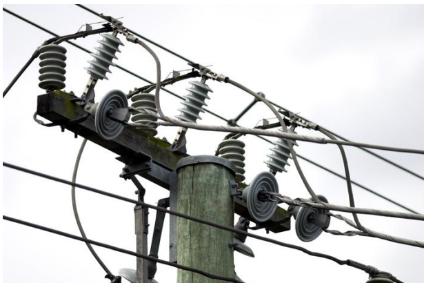
Examples of insulators
