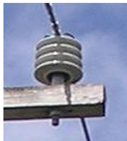
Low voltage insulator
