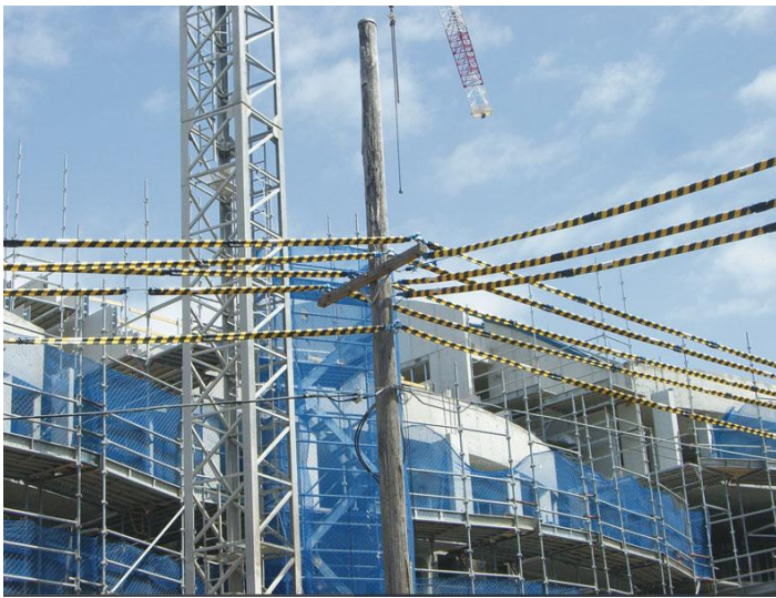
Tiger tails fitted over power lines near a construction site
