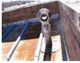
Asbestos cement roof vent pipe
