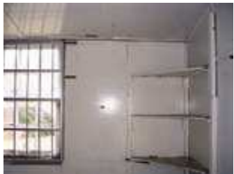
Asbestos cement wall lining
