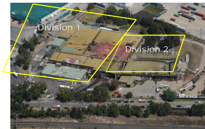
Figure 8 Divisions established at a large structure fire
