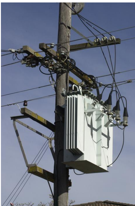
Pole-mounted substations
