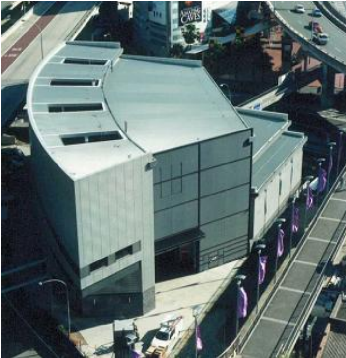
Enclosed zone substation – City Central at Darling Harbour
