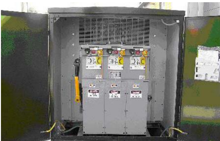
Internal view of a kiosk showing the high voltage end
