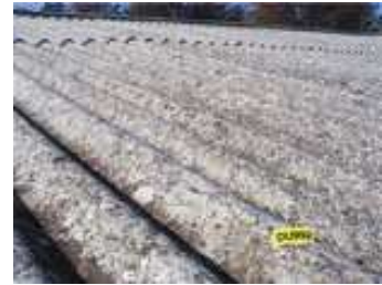
Corrugated asbestos cement roof
