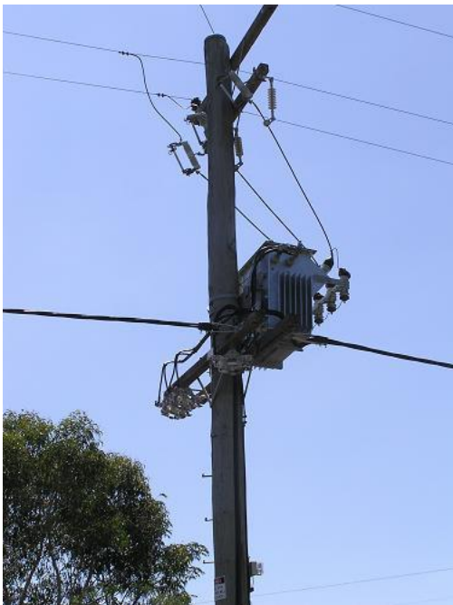
Pole-mounted substations
