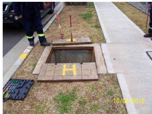
Figure 3 - Gatic® lifters used to open covers
