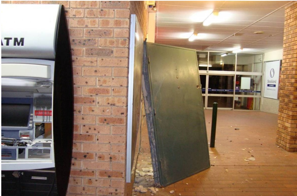
Figure 2 Door blown off hinges by force of explosion shown in Figure 1
