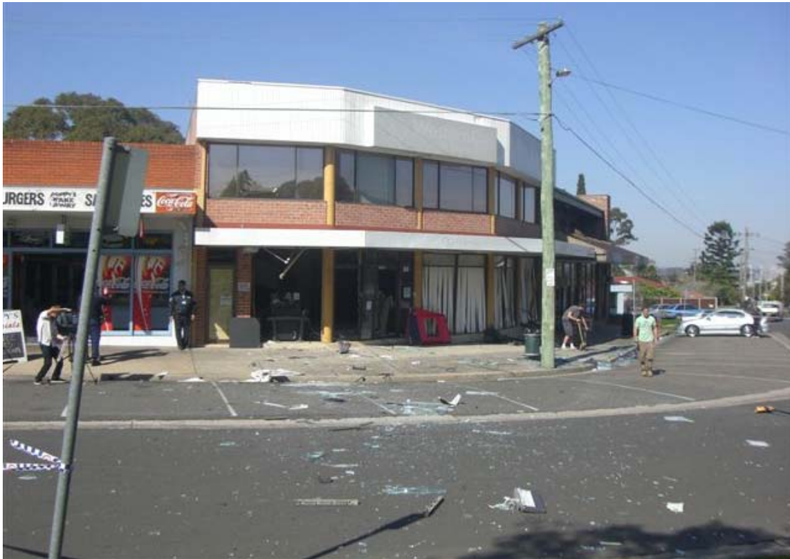
Figure 4 Shopfront destroyed by force of explosion
